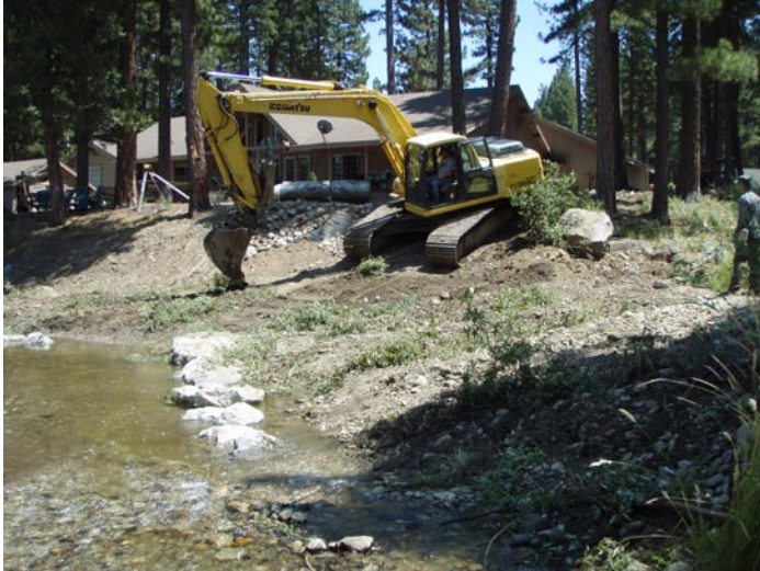
Photo on left: Construction of vanes on Smith Creek, Longnecker's bank.
